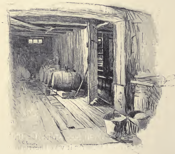
CELLAR AT THE PRESENT TIME IN THE MARSHALL HOUSE, SCHUYLERVILLE, WHICH WAS USED AS A HOSPITAL FOR THE BRITISH.
